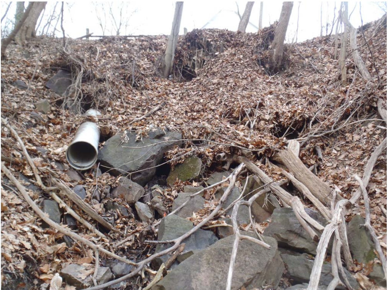
Photo 5: Large Stone Rip-Rap at Outfall
