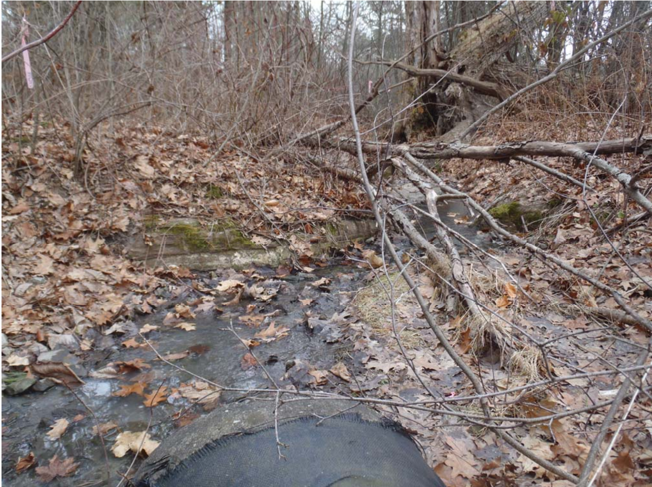
Photo 3: Looking Downstream from the 15" Concrete Pipe Outfall
